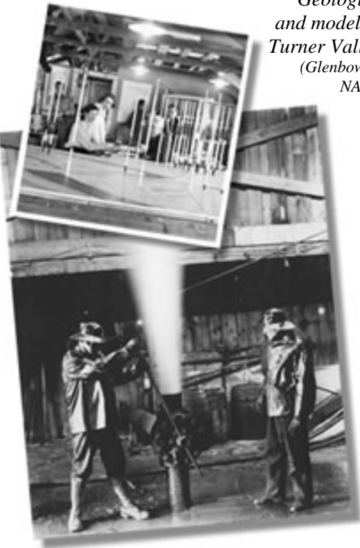
Blowing gas to reduce pressure at Turner Valley 1927 (Glenbow Archives ND-8-445)
