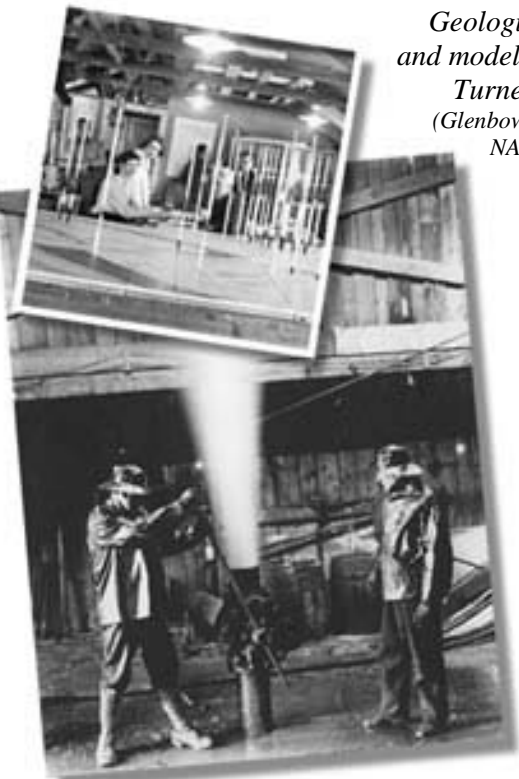
Blowing gas to reduce pressure at Turner Valley (Glenbow Archives NA-8-445)
