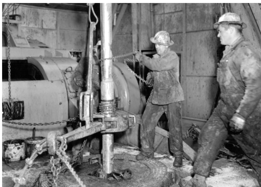
Drillers at work throwing the chain to make a connection, Western Canada circa 1960.
