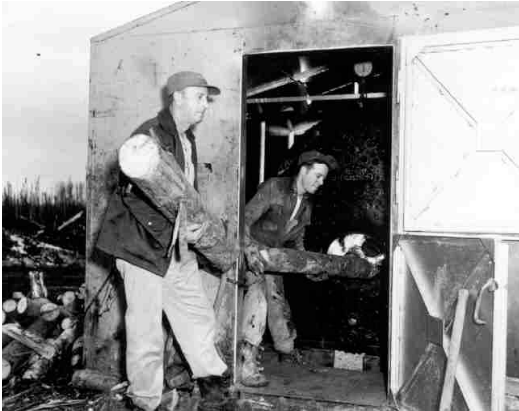
Well “logging” at Shell Klua Creek #1 in the 1950's. In these early days of drilling in northern Canada, the boilers on the rigs were commonly wood-fired and it was necessary to harvest the timber from a large area around the actual wellsite lease to provide enough firewood for the duration of the drilling program. Illustration courtesy of Shell Canada Photo Archives.
