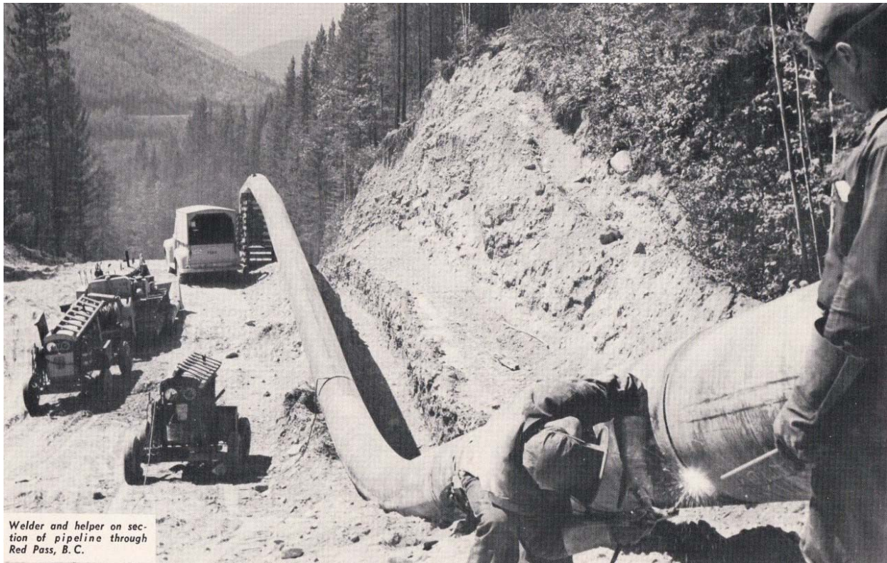
Pipe is strung along ditch ready for lining up and welding.
