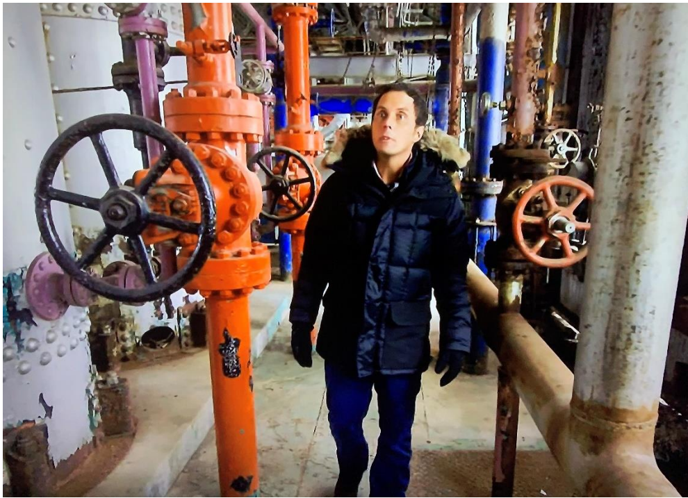
Jonny Harris inspects the piping in the sweetening building at the Turner Valley Gas Plant.
